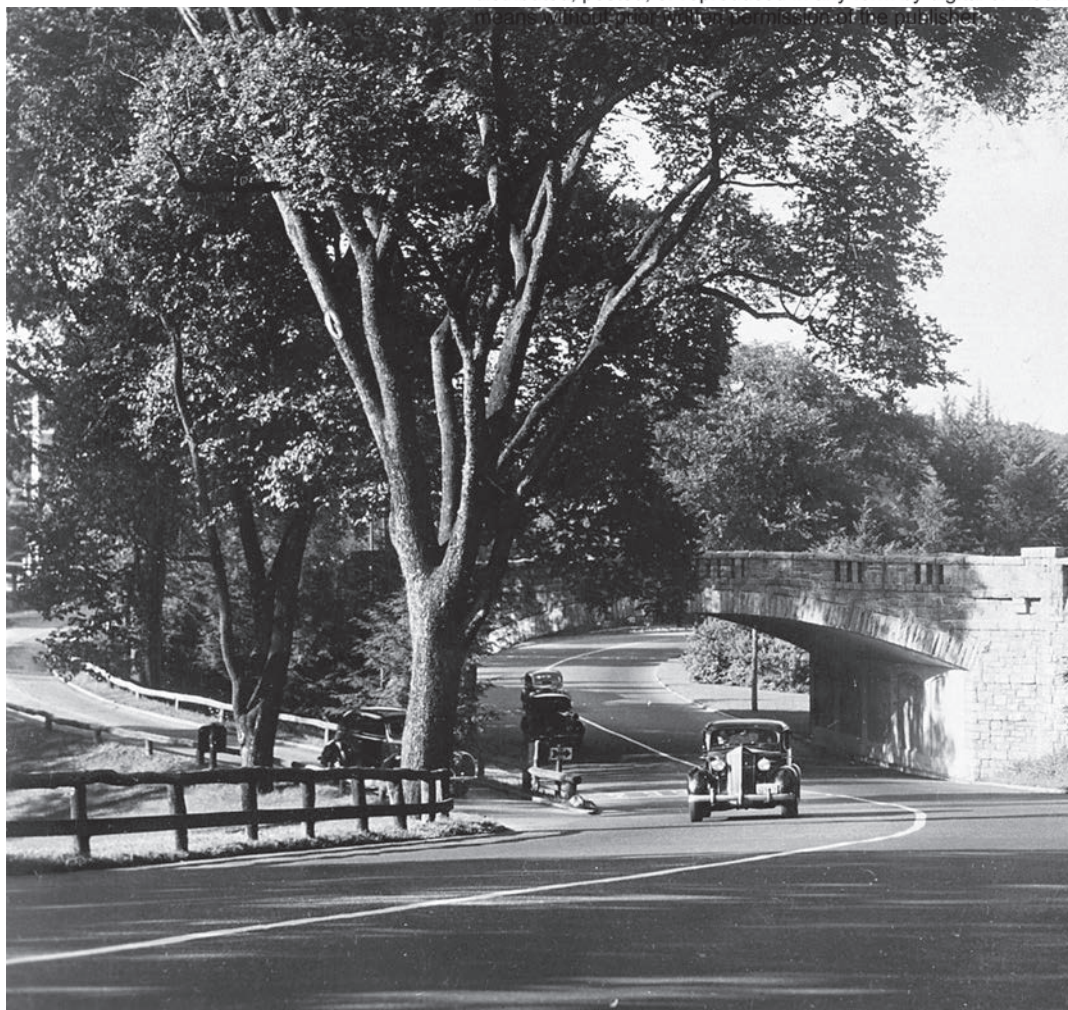
Bronx River Parkway, looking north to Fenimore Road overpass (demolished), ca. 1939. Westchester County Historical Society.
