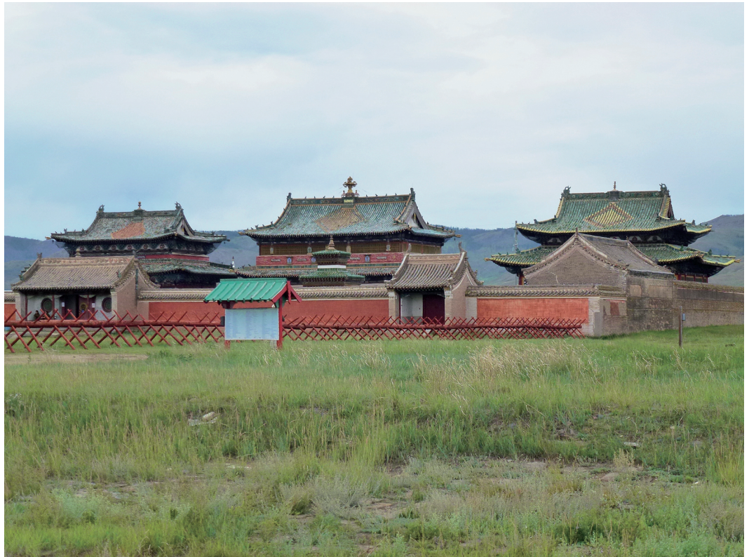
1.12 Tsogchin (Assembly Hall), Erdene Zuu, Khara-Khorum, Övörkhangai, eighteenth century with later repairs. Central of three buildings in photograph.
